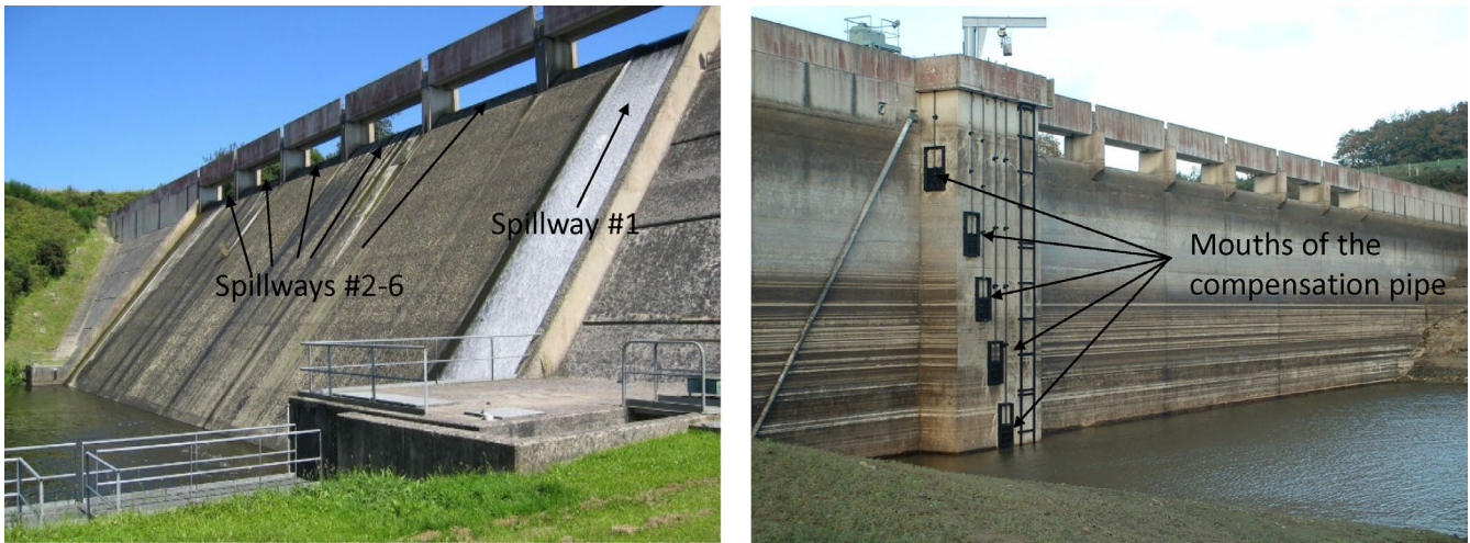
FIGURE 2 Details of the study site: Downstream view of the six spillways (left) and compensation pipe mouths during 10 years of draining (right). Spillway 1 is actively spilling water in the photograph
