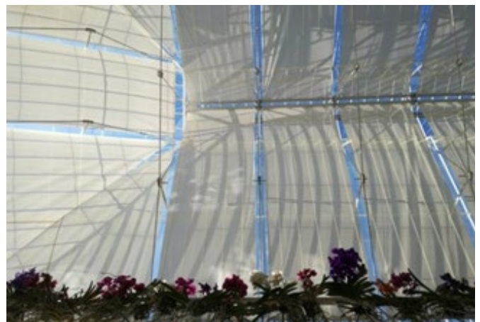
Figure 5: Automated ceiling screens
