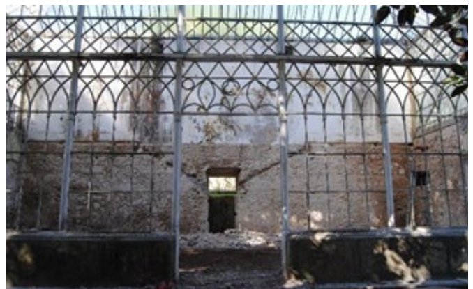
Figure 2: Restoration and rehabilitation
