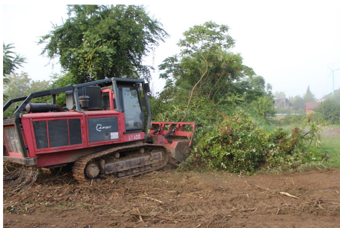
Figure 1: Cleaning the area with a mulcher
