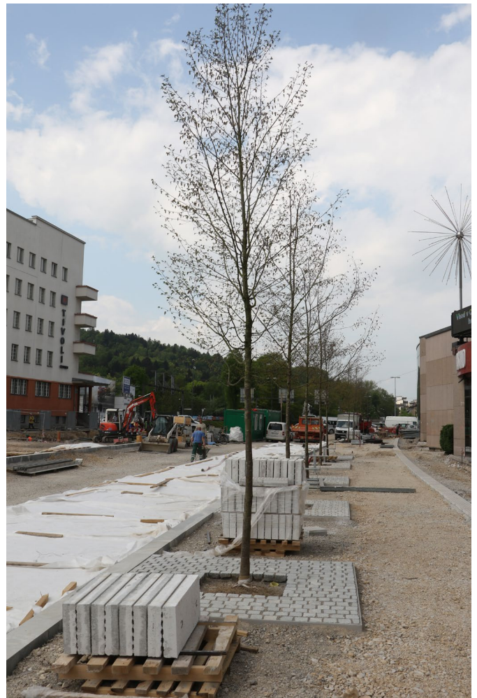
Figure 3: Last renovation of streets in Ljubljana in 2018
