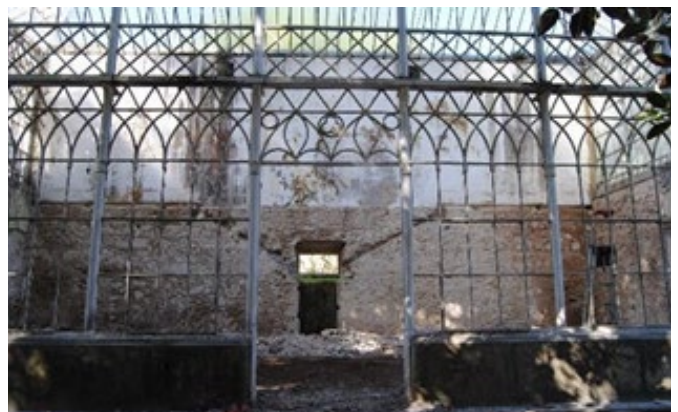
Figure 2: Restoration and rehabilitation
