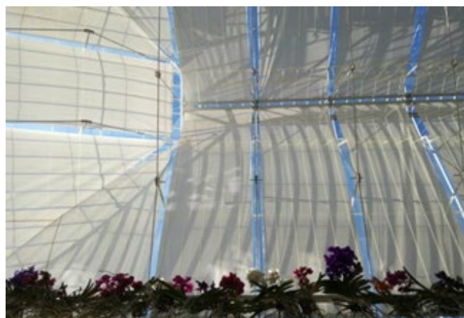
Figure 5: Automated ceiling screens
