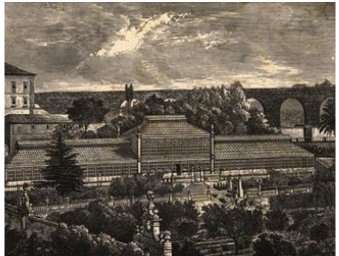
Figure 1: The newly built glasshouse in 1868
